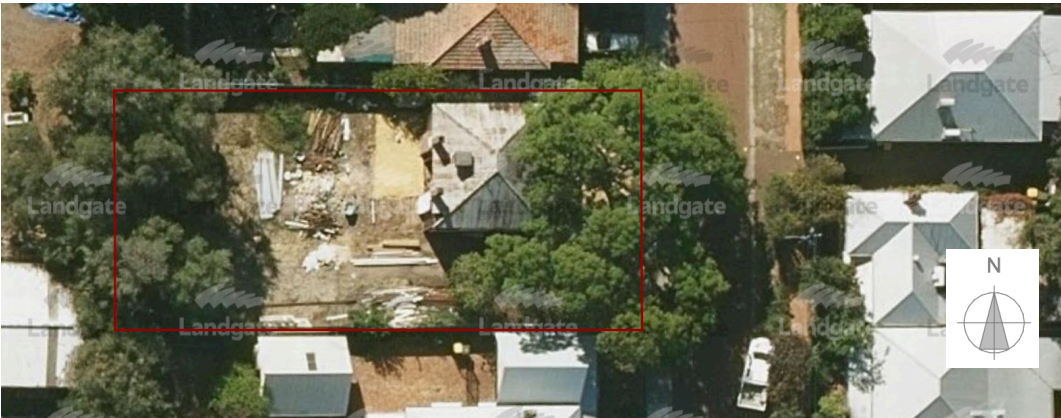
Figure 7. 2020 aerial photograph showing demolition (Landgate Historic Aerial Photograph).
