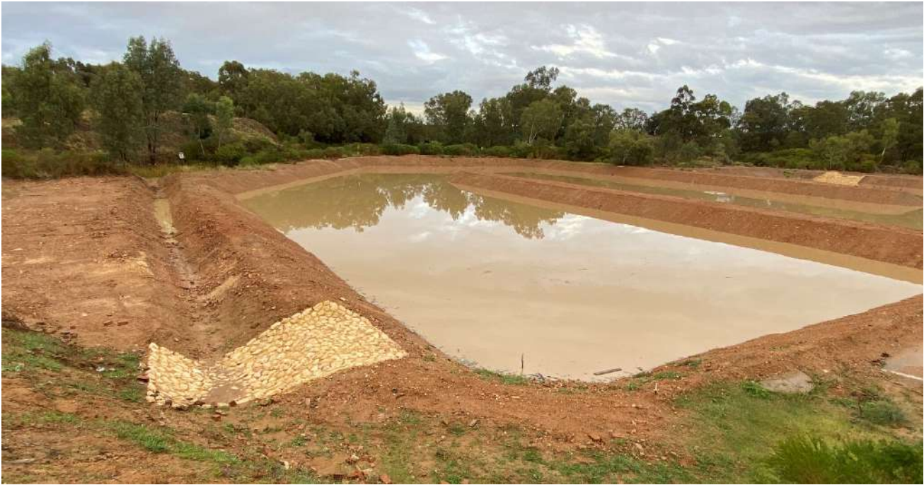
PLATE 17: Southern sedimentation storage area, main storage. (In process of decommissioning and relocation as part of Area 3 Stage 5 works)
