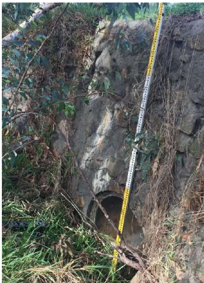
PLATE 10: 900 mm dia pipe under Muriel St. Invert of pipe is several metres below road level. Standing water will occur following events due to level of downstream pipework
