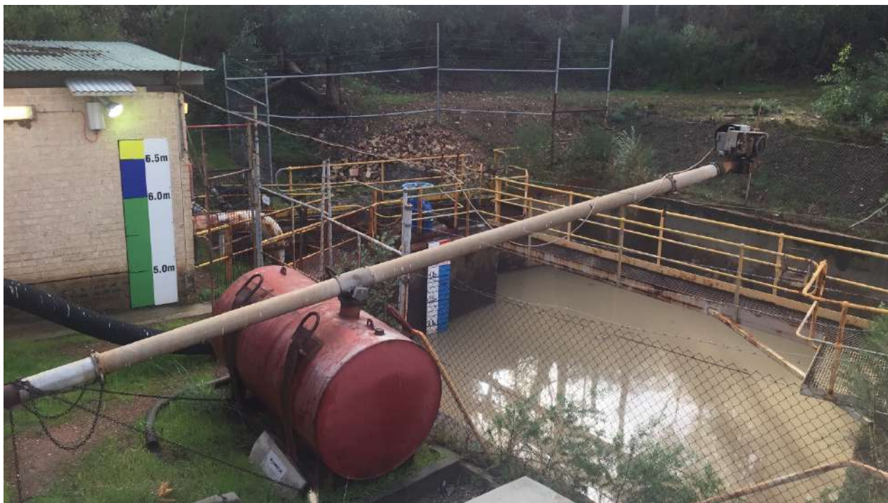
PLATE 11: Main Site Sump and Pump. Main Electric Pump (170 l/s) located in building
