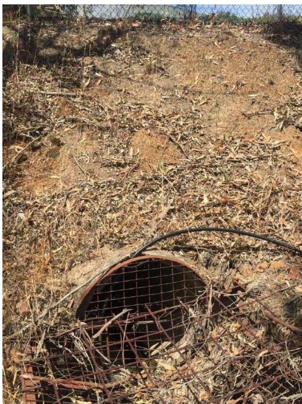
PLATE 16: Upstream end of existing outlet to Swan River near Clay Basin.
