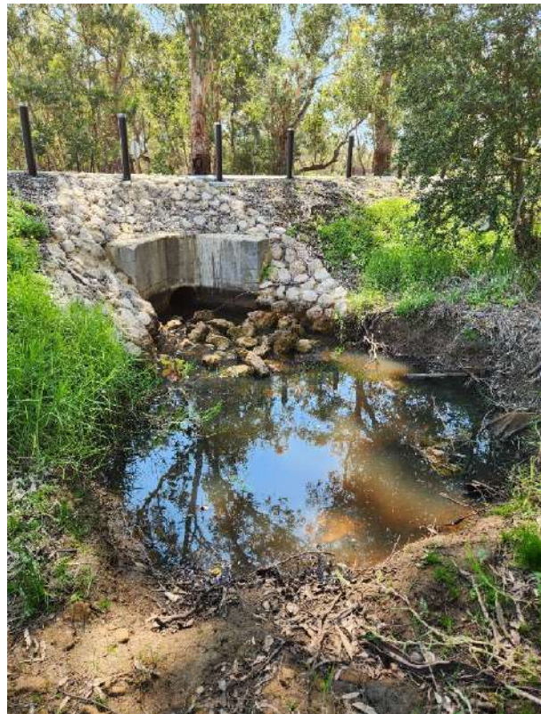
PLATE 4: Upstream and Downstream end of 450mm dia Culvert under Eveline Rd.
