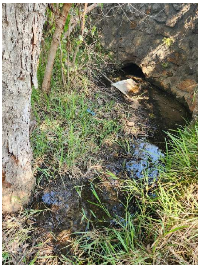
PLATE 10: 900 mm dia pipe under Muriel St. Invert of pipe is several metres below road level. Standing water will occur following events due to level of downstream pipework
