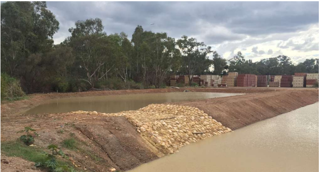
PLATE 18: Southern sedimentation storage area, forebay (In process of decommissioning and relocation as part of Area 3 Stage 5 works)
