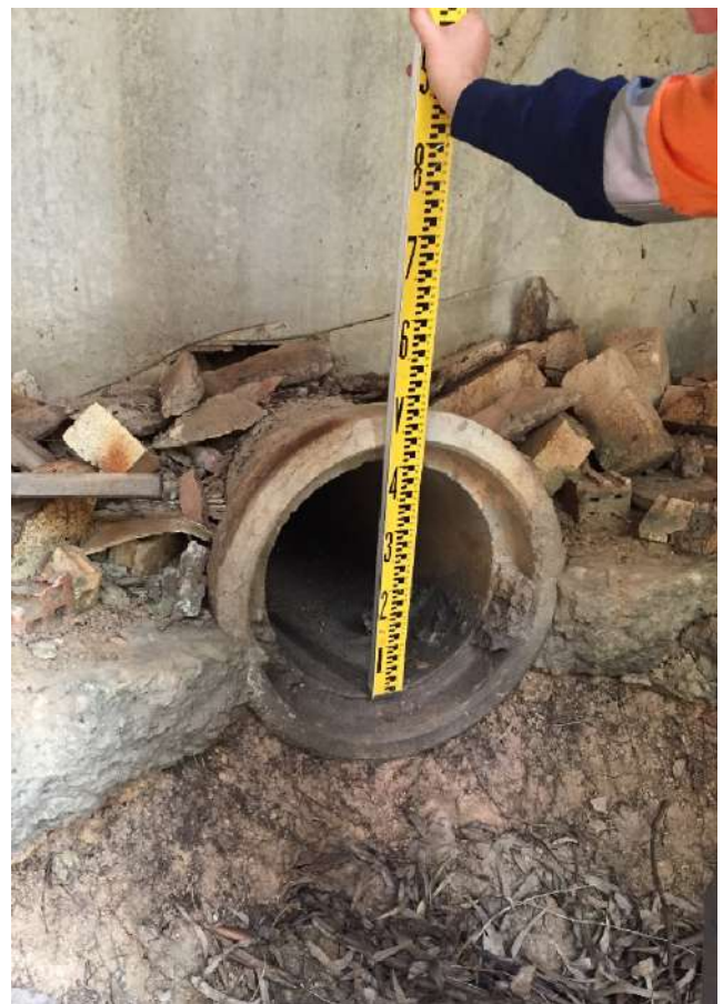
PLATE 21: 400 mm dia southern outlet upstream end in concrete tomb at end of open drain
