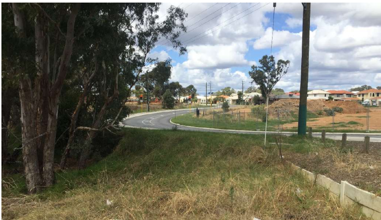
PLATE 9: Culvert under Muriel St at low point.
