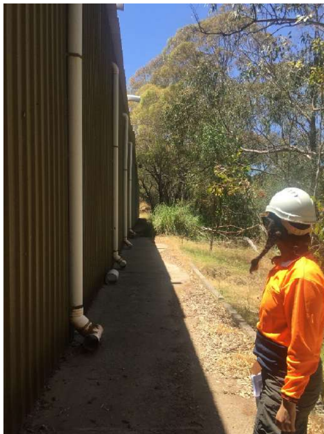
PLATE 13: Discharge from existing Clay Shed roof to storage area adjacent to TEC area
