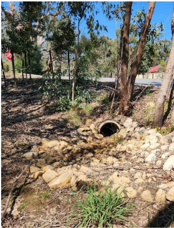
PLATE 4: Upstream and Downstream end of 450mm dia Culvert under Eveline Rd.
