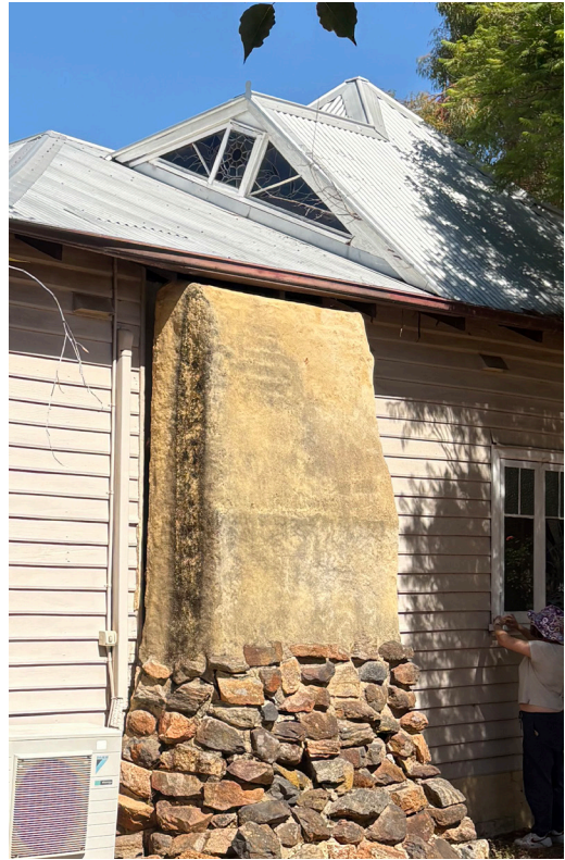
Figure 16. Detail showing chimney removed above roof line (DAR Studio, February 2026).
