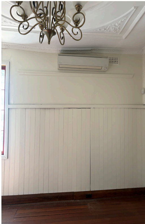
Figure 17. Interior, showing location of removed fireplace and mantle, closed with vertical timber boarding (DAR Studio, February 2026).
