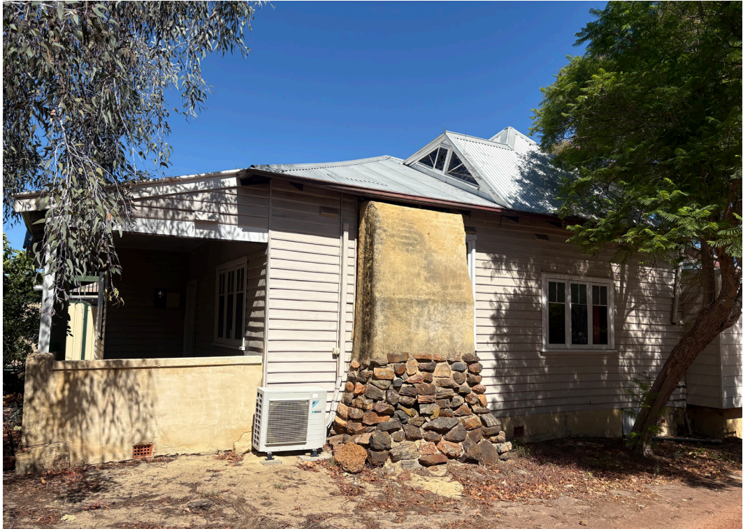
Figure 12. Side (north-east) elevation of residence, showing complex roof form, front verandah (dwarf wall proposed for removal), chimney (proposed for removal), and skylight above (proposed replacement) (DAR Studio, February 2026).
