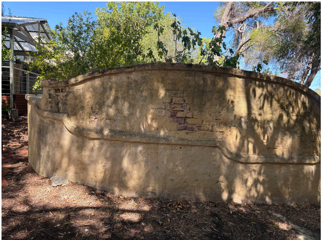
Figure 22. Side (north-east) of property, showing rendered brick wall, proposed for removal (DAR Studio, February 2026).
