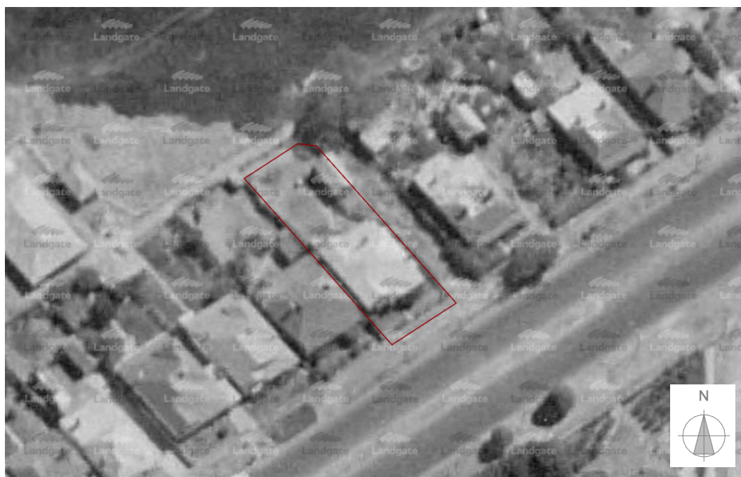
Figure 7. 1965 aerial photograph showing residence and detached garage to the rear (Landgate Historic Aerial Photograph).
