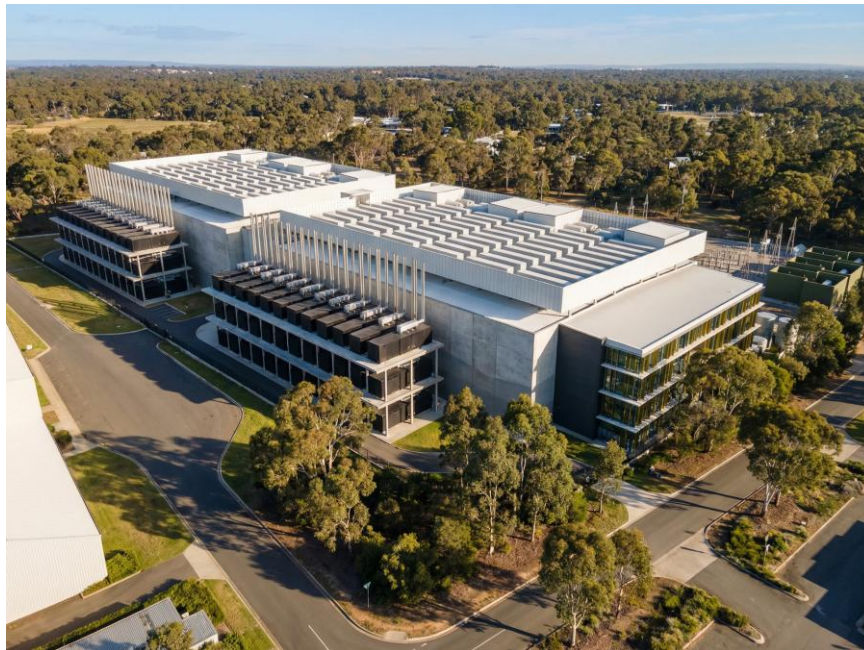
Figure 13 Aerial View of Data centre.
