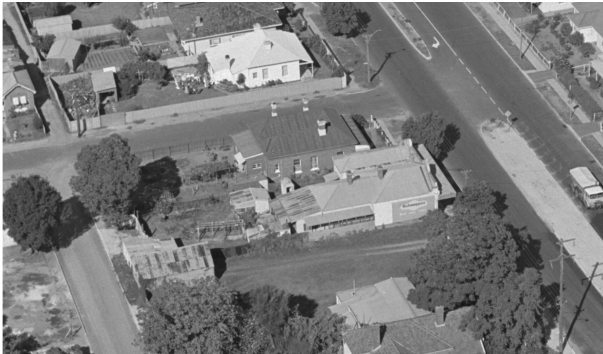
Figure 5. Looking south across the rear of No. 62 East Street, 1976, noting the timber picket fencing along Turton Street (Extract from SLWA 361876PD)
