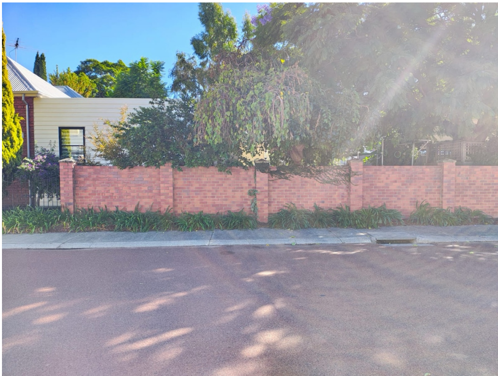
Figure 12. View looking north in Turton Street towards the existing solid wall forming the secondary street fence towards the rear of the lot. (Element Advisory, 2026)
