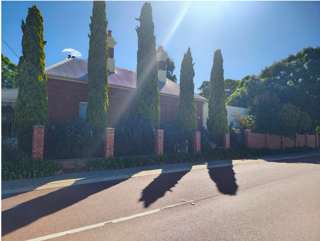
Figure 11. The fence and wall along Turton Street constructed in c.2003 which is to remain as existing, with views to the dwelling retained. (Element Advisory, 2026)
