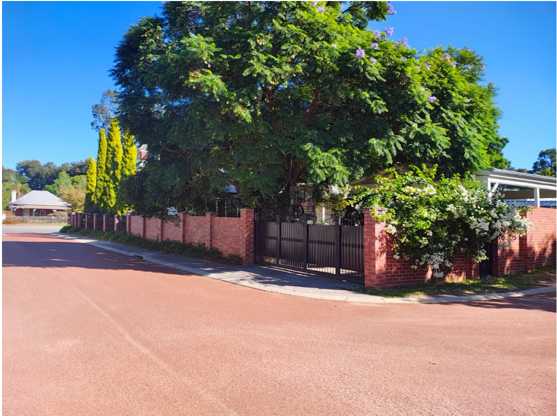
Figure 15. Looking north-west in Turton Street, near the intersection of Gibbons Avenue, towards the subject site and showing the full secondary street fence, wall and vehicle access gate. It progresses from visually permeable where views of the dwelling contribute to the streetscape closer to East Street to a solid treatment at the rear of the lot. (Element Advisory, 2026)
