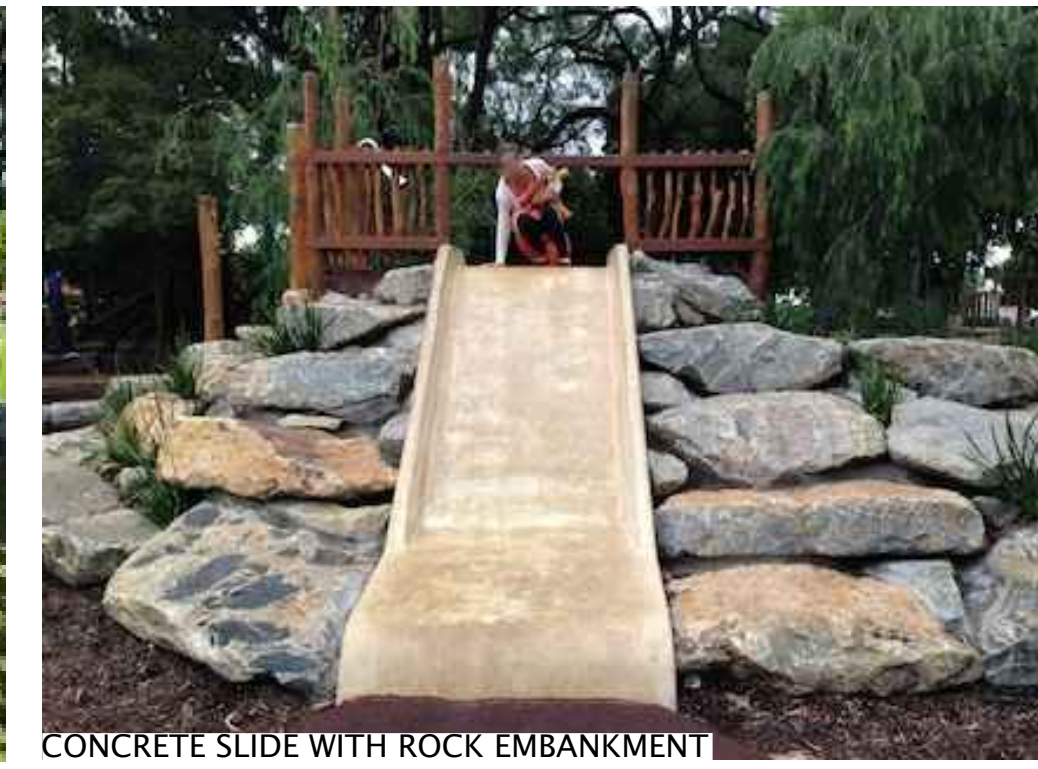
CONCRETE SLIDE WITH ROCK EMBANKMENT
