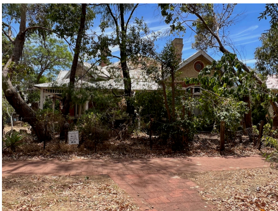
January 2023: Front (south) elevation of 112a Helena Street.
