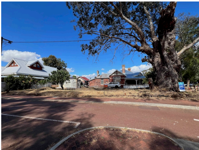
November 2025: View to northeast in Stephen Street showing the secondary frontage of the subject site.
