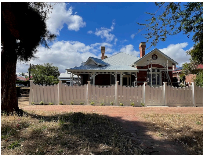
November 2025: South (front) elevation of residence at 112a Helena Street.
