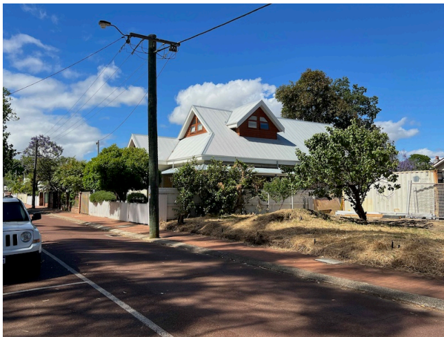
November 2025: Views to northeast in Stephen Street showing the secondary frontage of the subject site.
