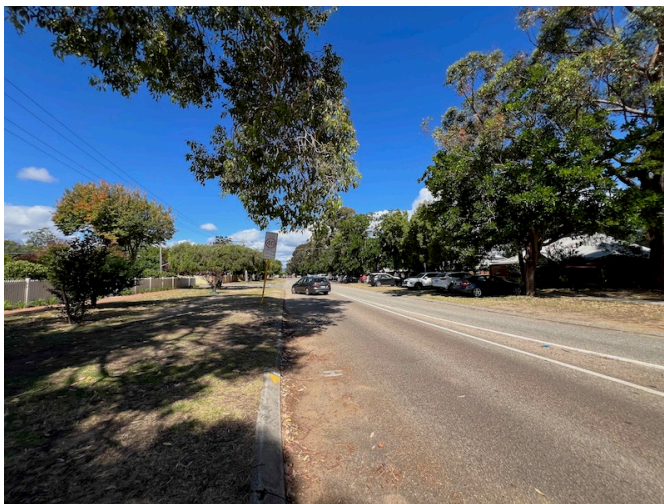
November 2025: Views from the roundabout looking southeast to school, and east in Helena Street.
