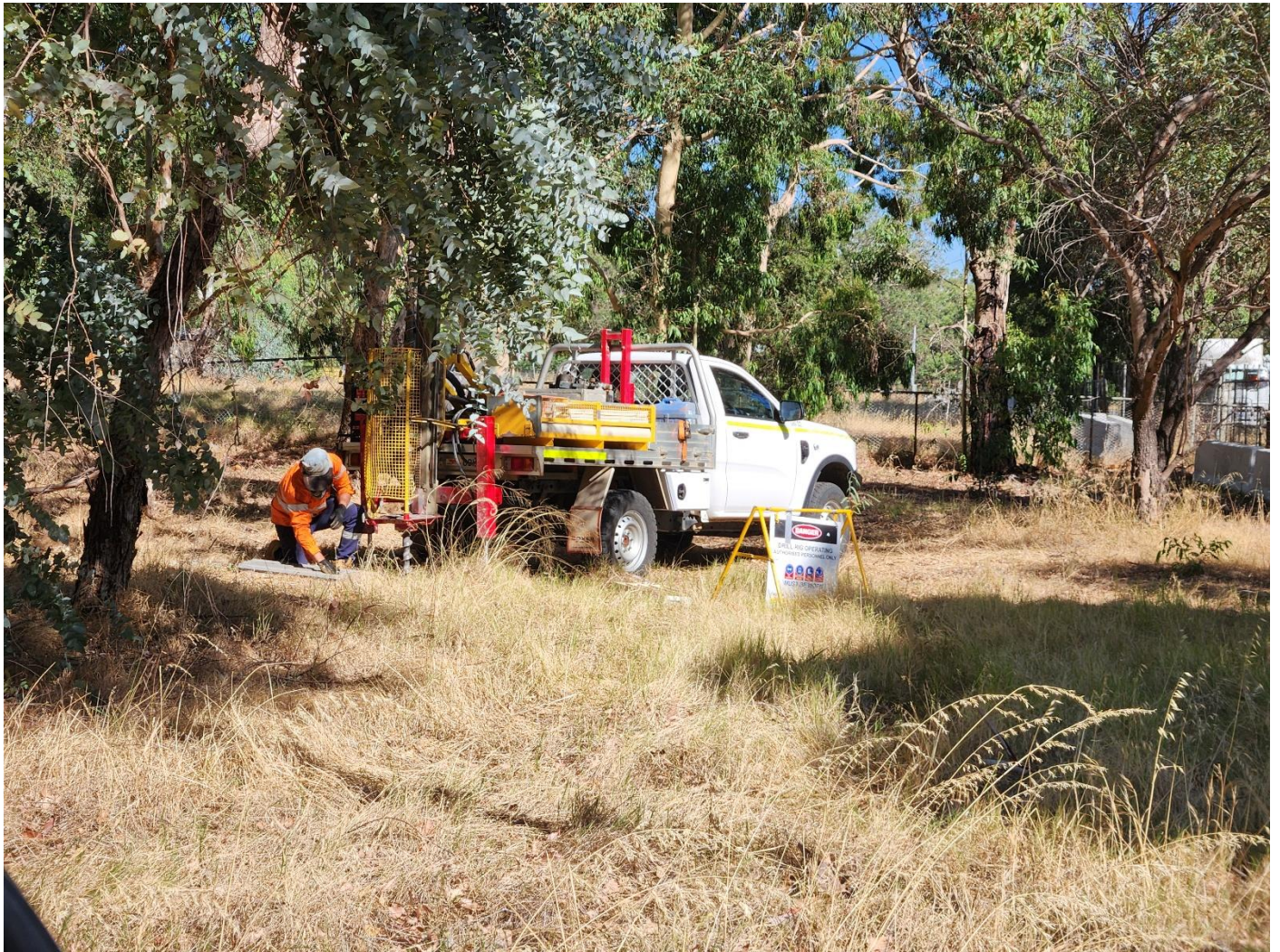
Photograph 6: Facing northwest at BH05 location. BH05 in progress.
