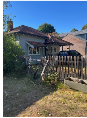
Fig 10. #6 Meares St Gable wall
