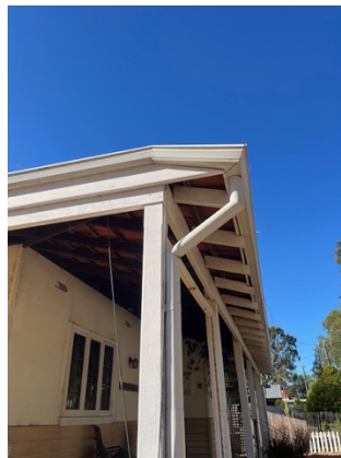
Fig 8. Verandah – existing eaves (WDG 17/3/2026)
