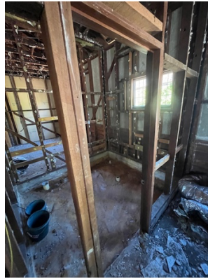
Fig 7. Current Bathroom (WDG 17/3/202)
