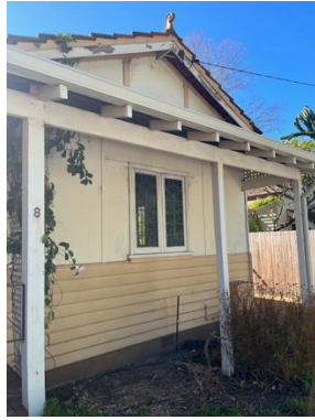
Fig 9. Gable Wall (WDG 17/3/2026)
