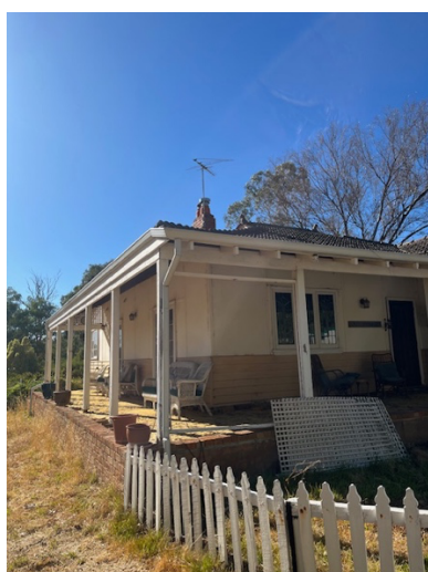
Fig.14 Verandah Retaining Wall (WDG 17/3/2026).
