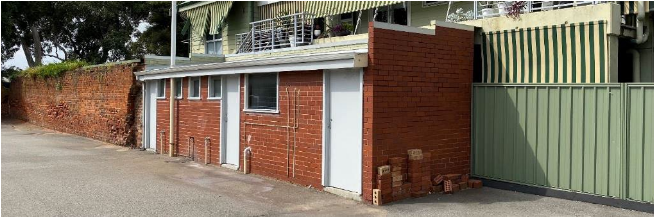
Figure 3 – Small external brick building on eastern boundary to be removed (Source: TBB, 2023).
