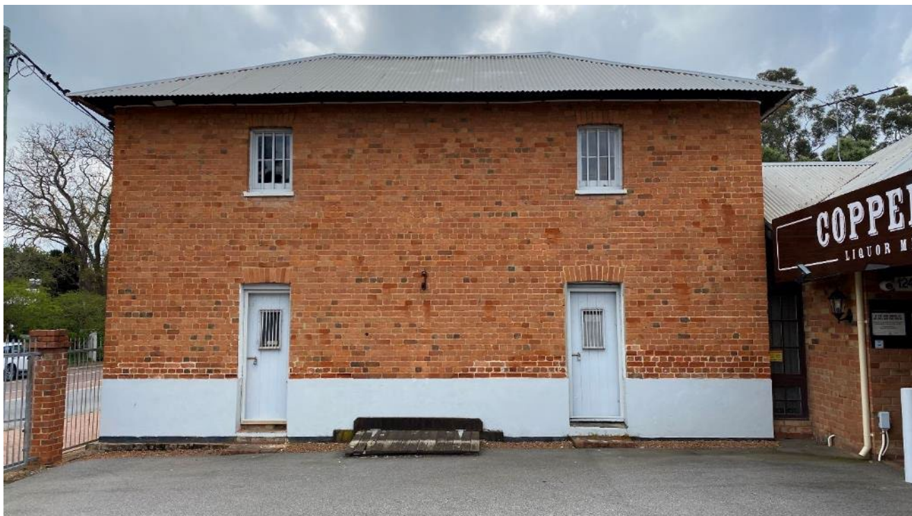
Figure 13 – Existing heritage building, looking north (Source: TBB, 2023).
