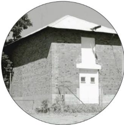
The proposal seeks to retain and rejuvenate the existing Baker's Warehouse and integrate this with the proposed fresh food market.
