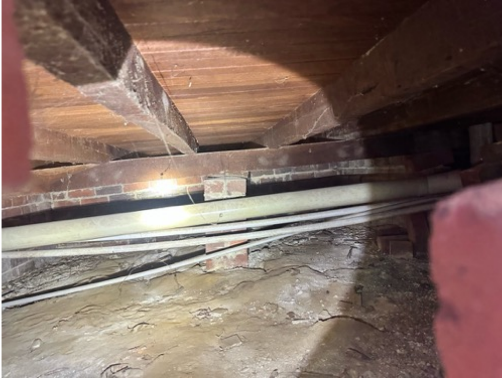
Missing bricks poor support to the west wall of the Dining room
