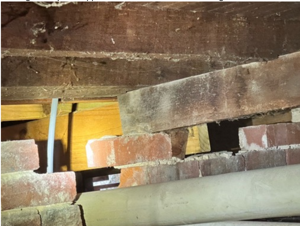
Missing bricks poor support to the west wall of the Dining room
