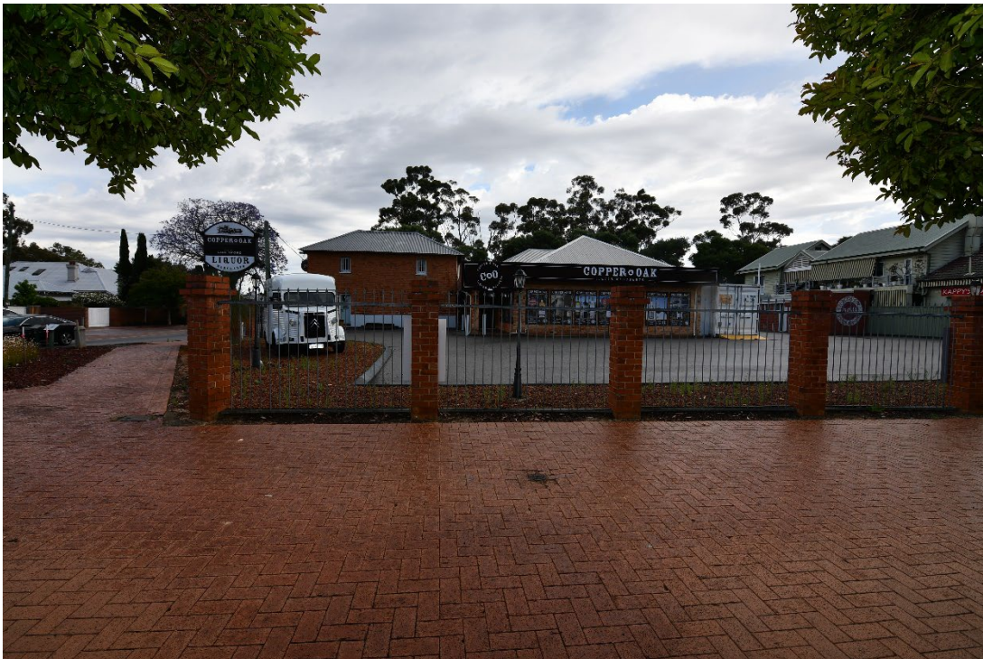
Photograph 04: View looking north towards 124 Swan Street from the corner of Swan and Meadow streets. Double-storey warehouse and more recent bottle shop visible behind fencing. Griffiths Architects, November 2024.
