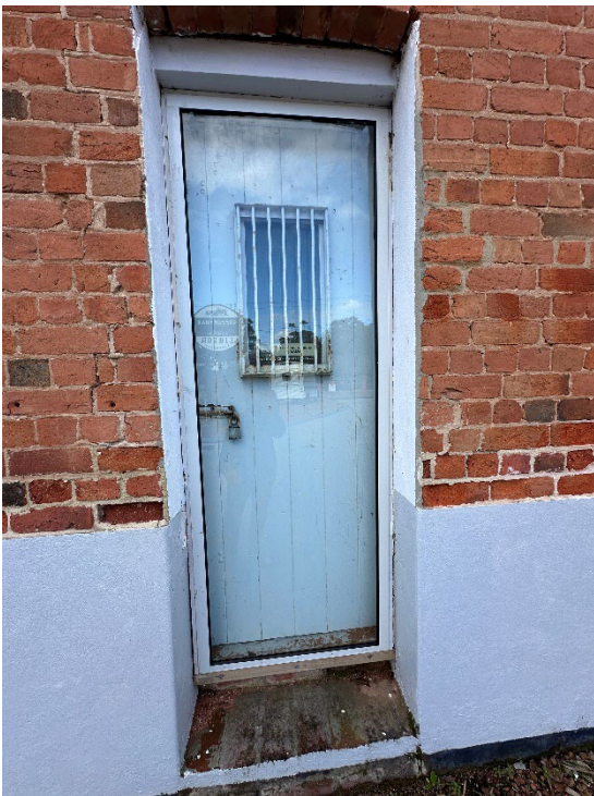
Photograph 16: Photograph showing the existing condition of the original access door to the double-storey warehouse. Griffiths Architects, August 2024.
