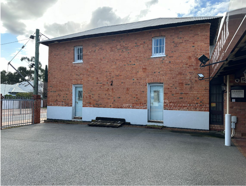
Photograph 11: View looking north toward the southern elevation of the double-storey warehouse. External hatch door to cellar/basement visible.. Griffiths Architects, August 2024.
