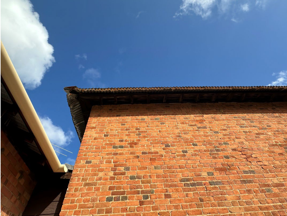
Photograph 13: Photograph showing the existing condition of the northern masonry wall band of the double-storey warehouse. Existing roof sheeting visible. Griffiths Architects, August 2024.
