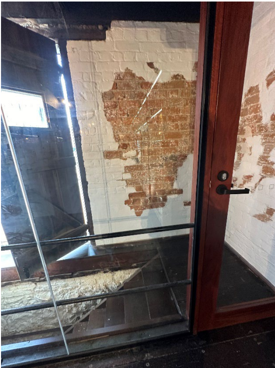
Photograph 18: Internal view showing access stairs to cellar. Stairs behind glazed wall. Griffiths Architects, August 2024.
