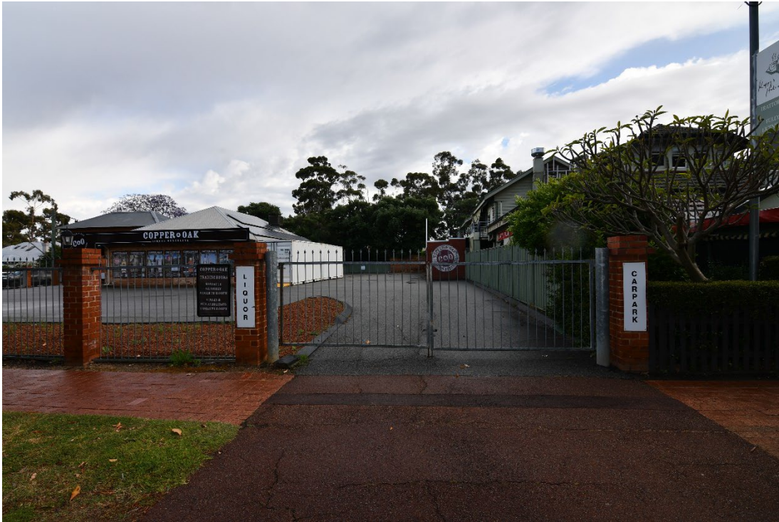
Photograph 05: View looking north towards vehicle access gate of 124 Swan Street. Griffiths Architects, November 2024.
