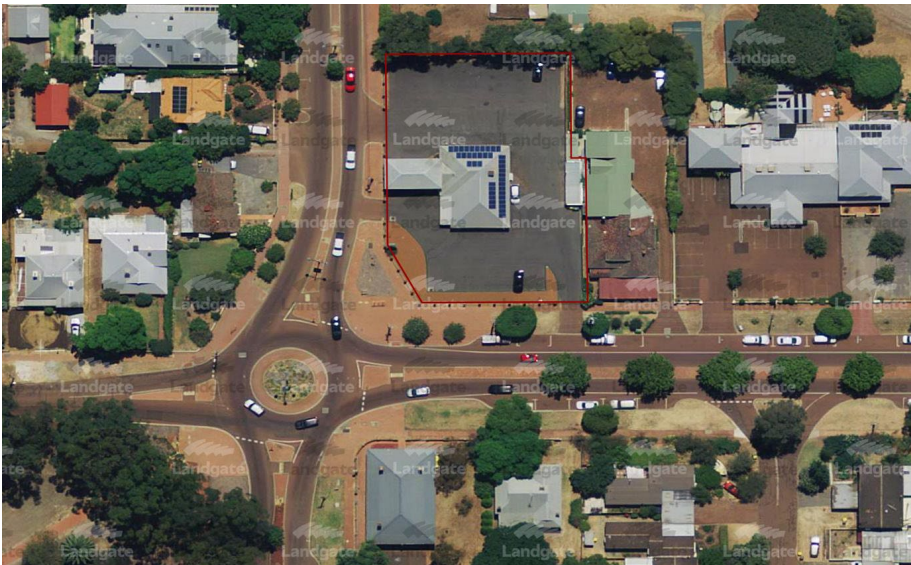
Figure 10: February 2014 aerial photograph showing the installation of solar panels atop the latter building at 124 Swan Street. Courtesy Landgate, 2024.
