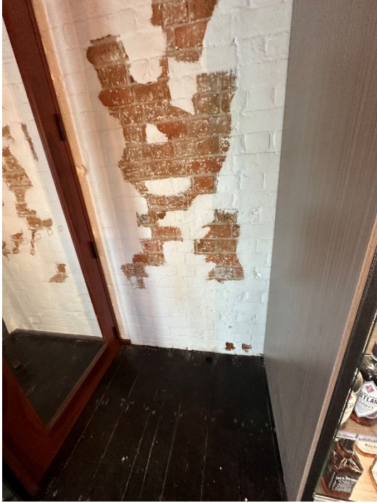
Photograph 17: Internal view showing condition of internal walls within the double-storey warehouse. Griffiths Architects, August 2024.
