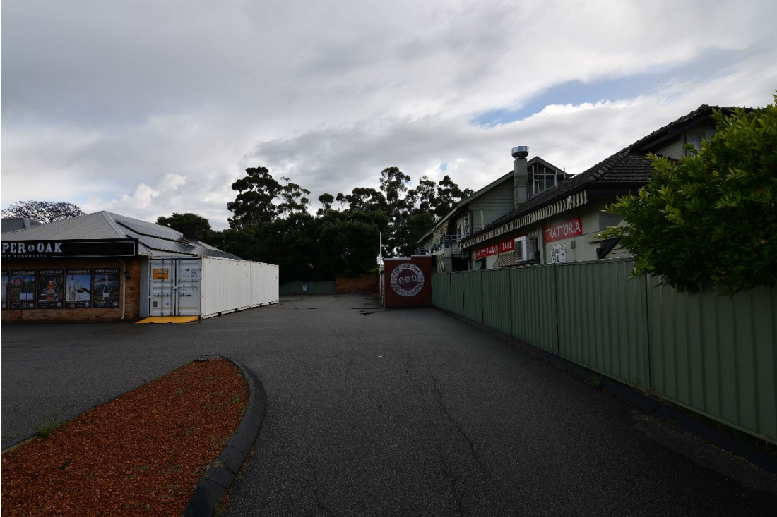
Photograph 07: View looking north showing subject site at 124 Swan Street, noting the smaller masonry structure along the eastern site boundary and large amount of bitumen coverage. Griffiths Architects, November 2024.
