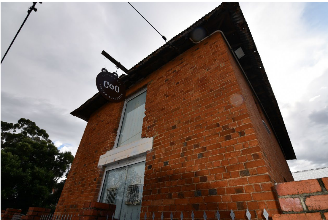
Photograph 06: View looking north-east toward the west elevation of the double-storey warehouse. Branded signage hung from former hoist visible. Griffiths Architects, November 2024.
